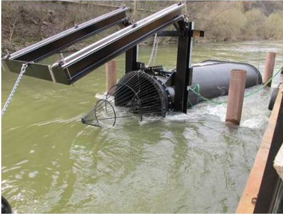
Figure 6. The River-Turbine prototype during installation. Source: KSB 2010. © KSB Aktiengesellschaft (2010)
