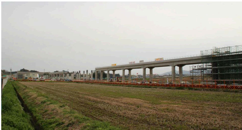
Figure 5 Jōban Railway Line construction site in Shinsakamoto in April 2015.
