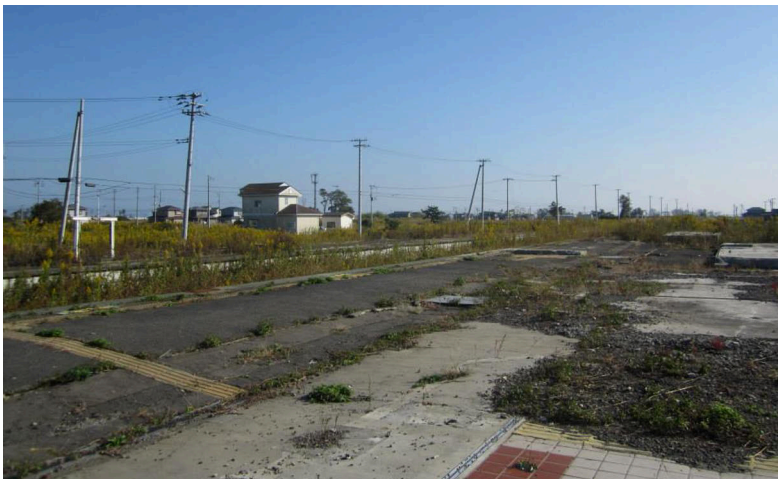
Figure 3 The platform of the now-demolished Yamashita station in October 2014.
