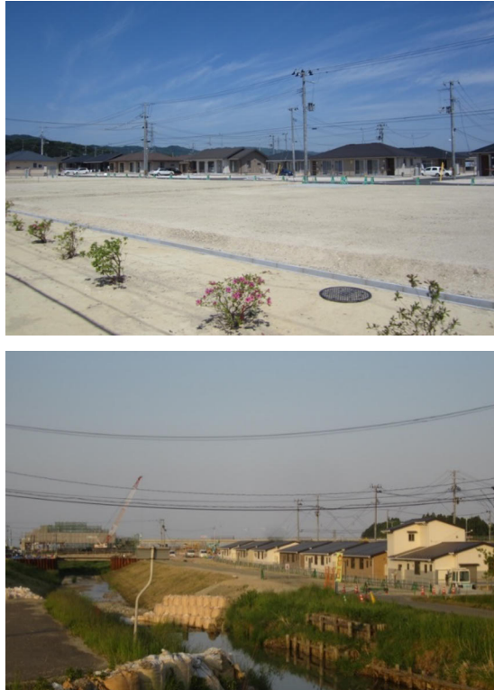
Figure 7 Compact city construction sites of Shinyamashita (above) and Shinsakamoto (below).
