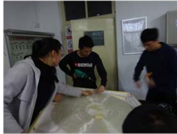
v. Installing tube
