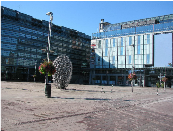
Figure 4. Kamppi Shopping Centre (looking from Narinkka Square southwards)
