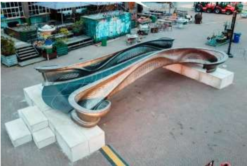
Figure 11 MX3D bridge created with WAAM [6]
